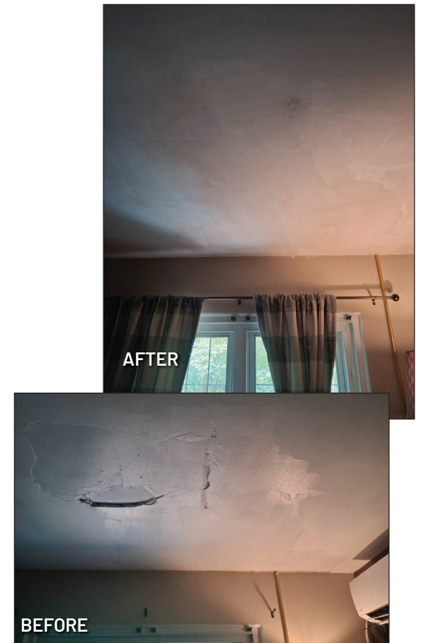
Building 813/1658 Ceiling Plaster Repairs
