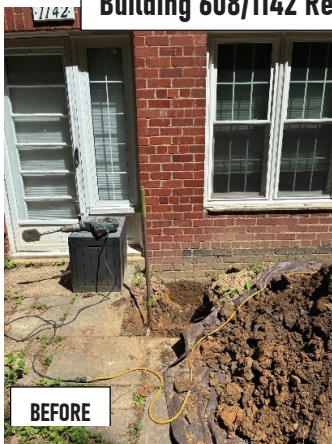
Building 608/1142 Rear Hydrant Installation
