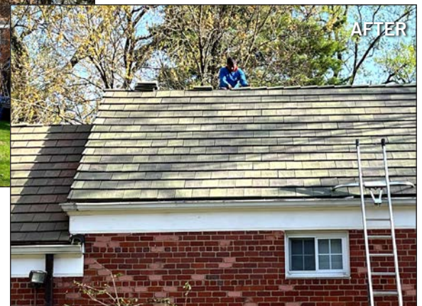
Building 510 Roof Replacement
