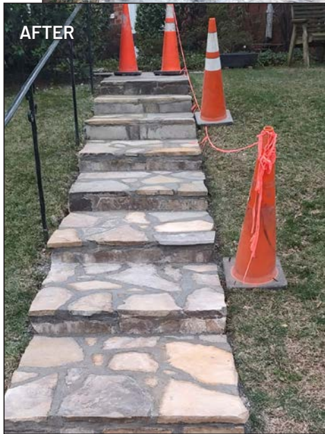
Building 202 Flagstone Repair
