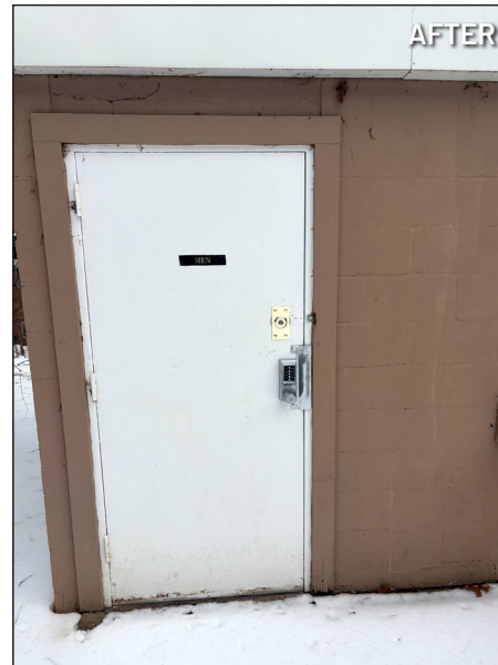
Valley Drive Tennis Court: Restroom Security Lock Installed
