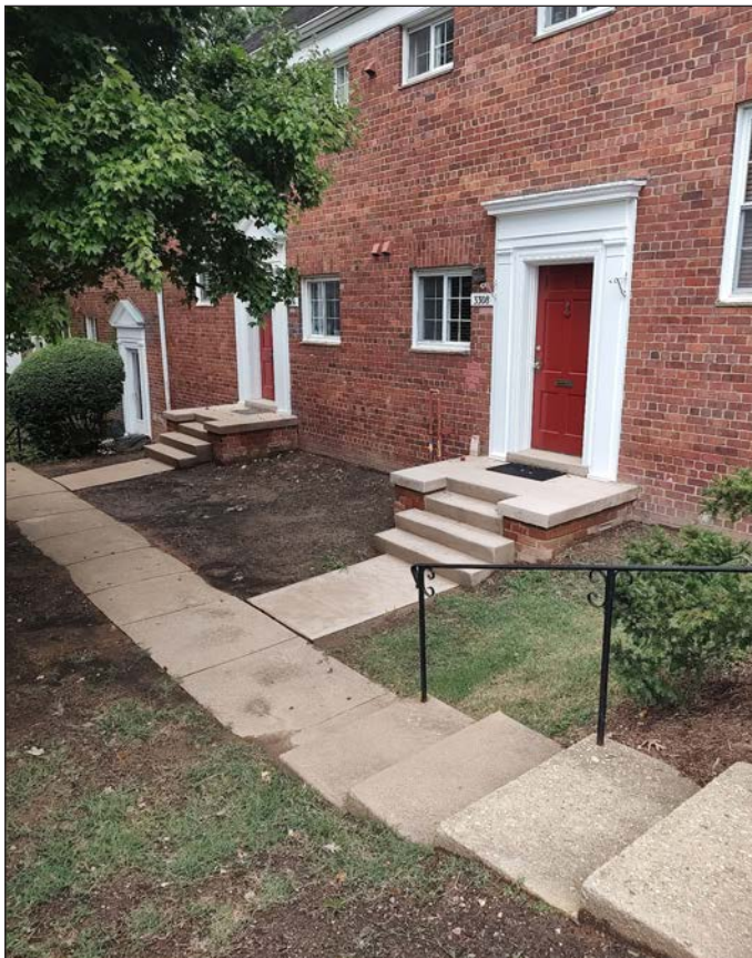
Building 728/3306 and 3308 Stoop Replacement
