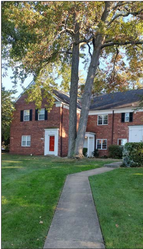
Building 602: Shutter Replacements
