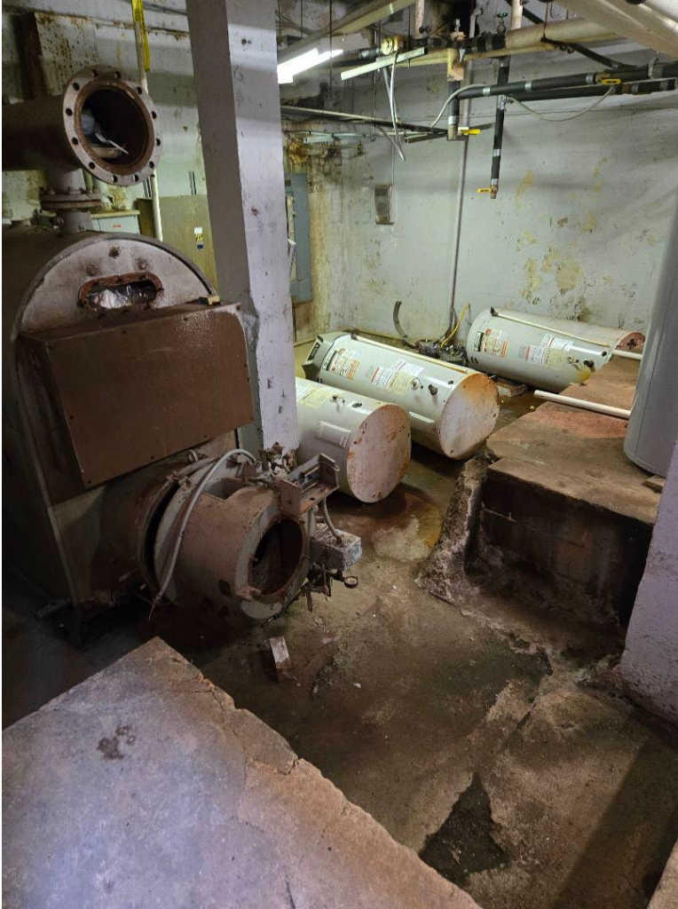
Appendix Photo 3: Disconnected water heaters staged on boiler room floor.
