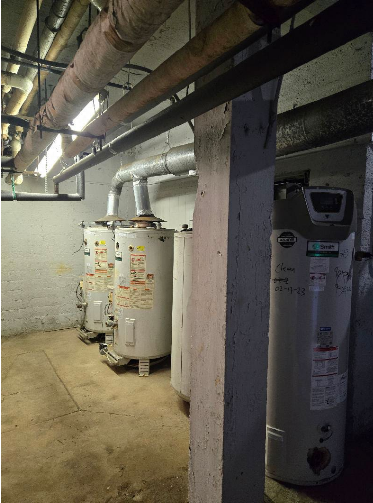
Appendix Photo 1: Connected A.O. Smith water heaters (set 1).
