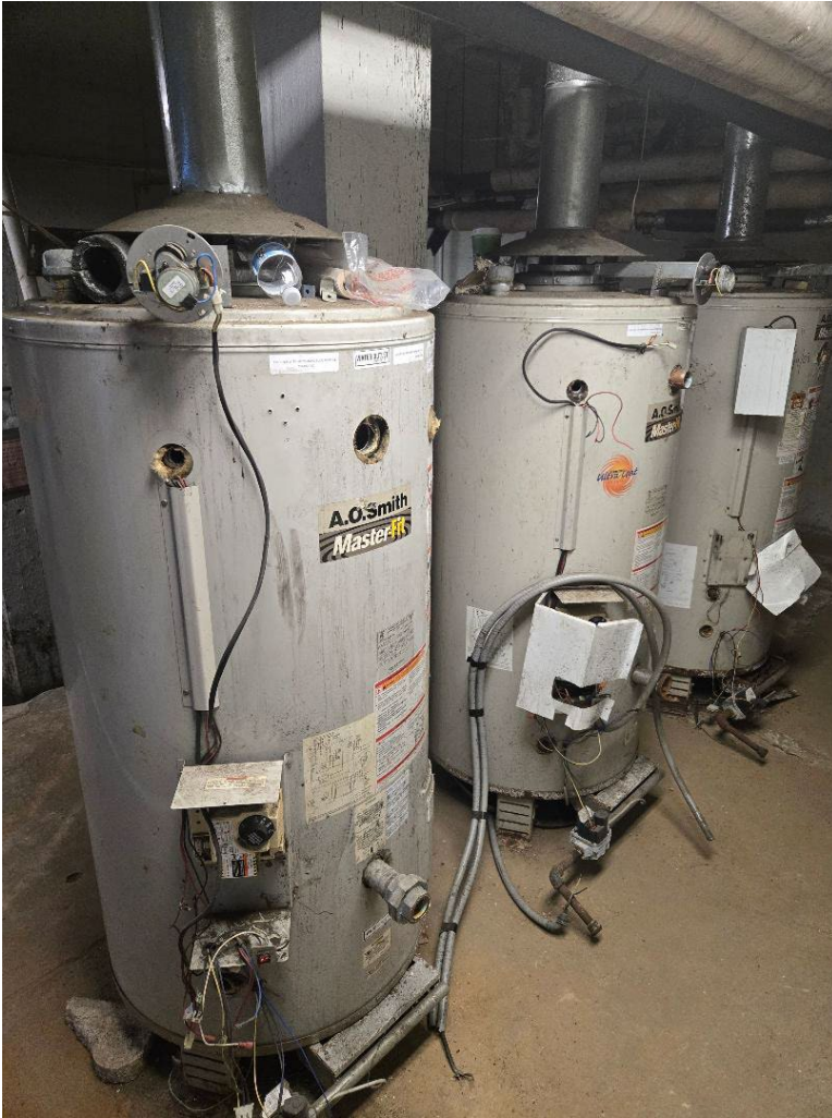
Appendix Photo 2: Connected A.O. Smith water heaters (set 2).
