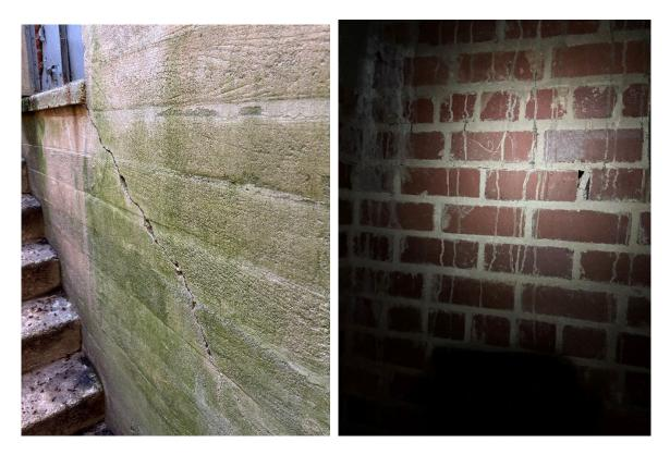
Based on our limited visual assessment while we were on-site, it appears there is moisture intrusion into the attic space due to the movement of the roof assembly and the cracks observed in the unit and crawl space appear to be due to differential settlement. There is the possibility that the movement of the roof assembly is related to the differential settlement of the building.
