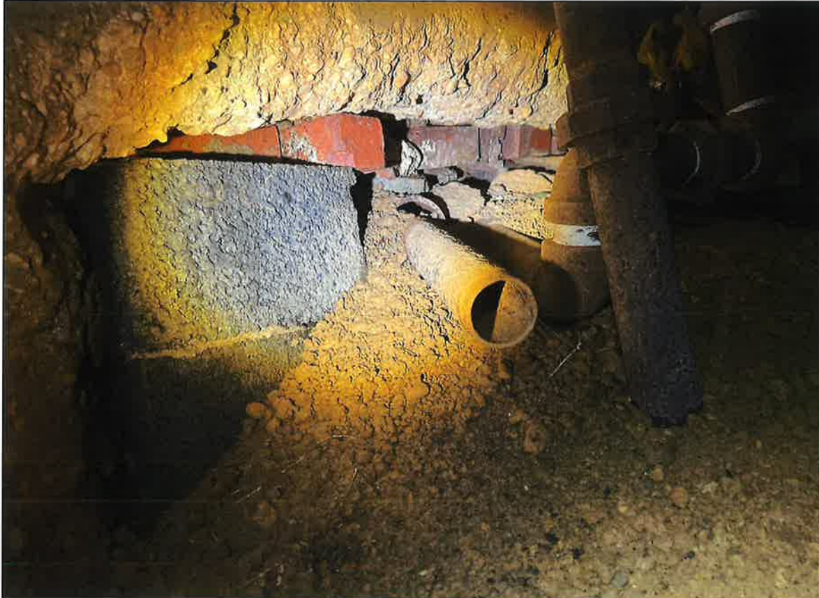
Photo 1. Demolished foundation wall at the rear of Unit 1670's foundation wall.
