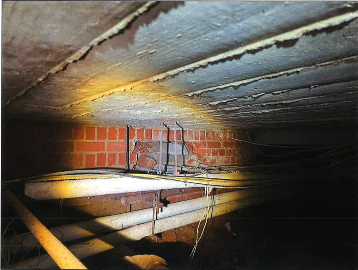
Photo 3. Opening in the side elevation foundation wall.
