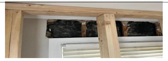
The brick lintel is a structural member. Given the age of the building, it doesn't meet today's requirements for a brick lintel.
