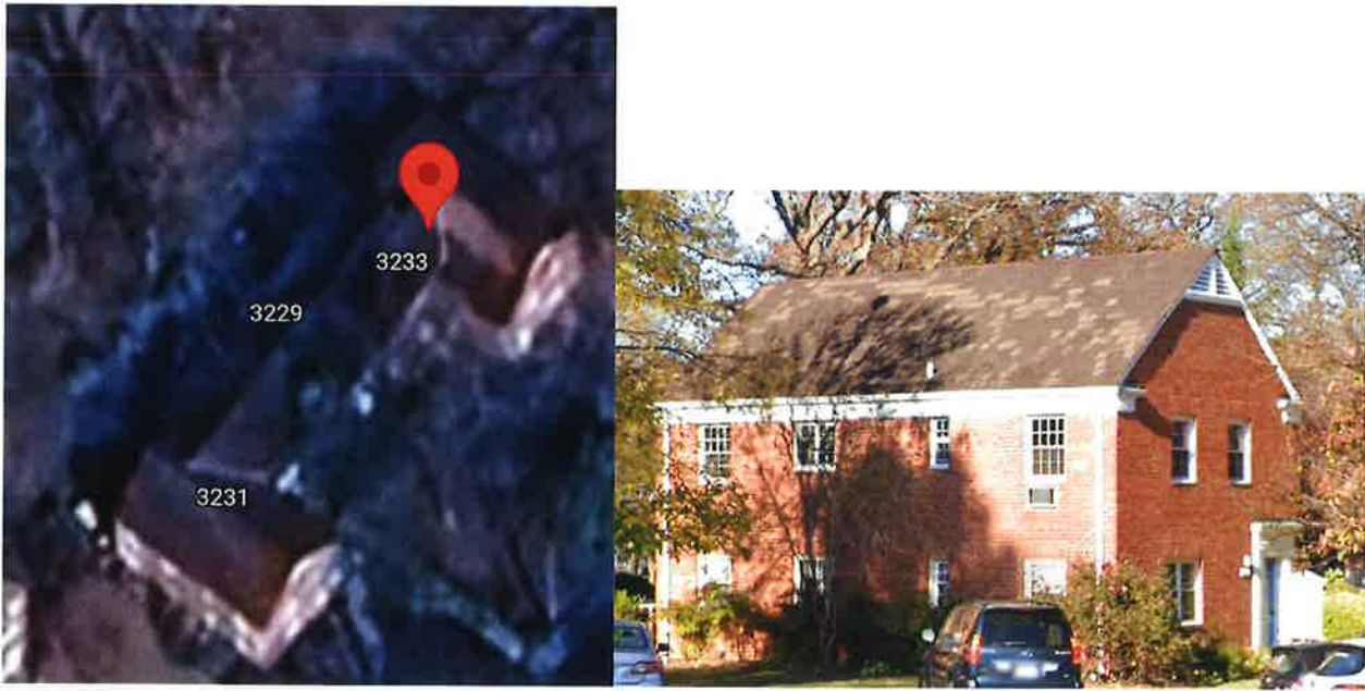
Figure 3: Building 849 Google Maps Images
