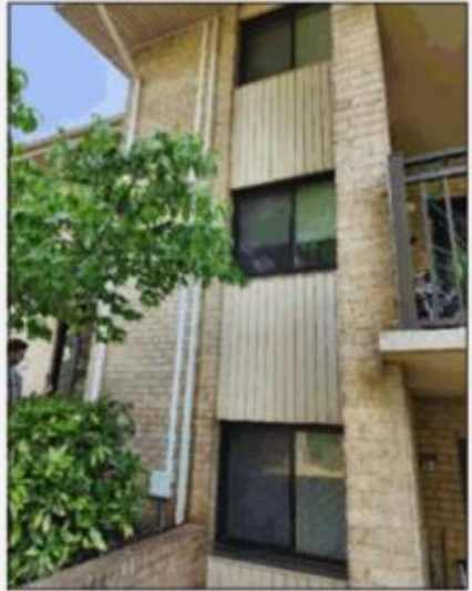
TYPICAL OF METAL MOLDING IN USE
