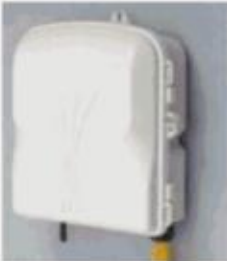
TYPICAL FIBER TERMINAL SIZE: 14.5" W x 16.2" L x 6" D
