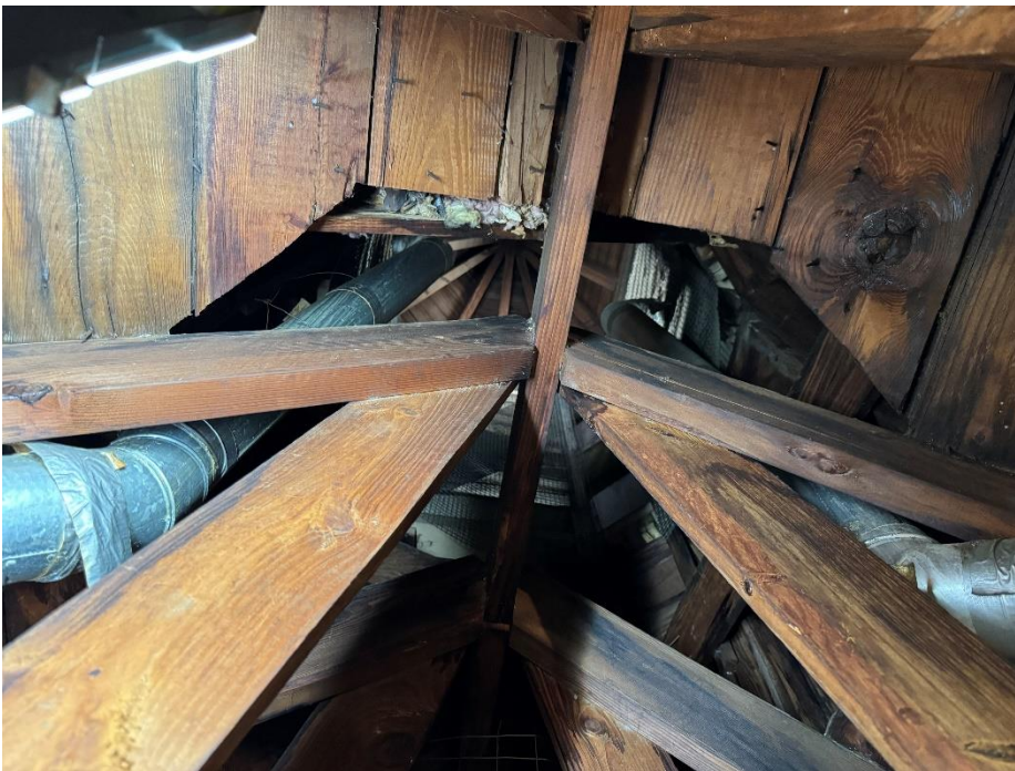
Photo 16. Bldg. 953: Cupola provides air flow for the attics of Units 1500 and 1501.
