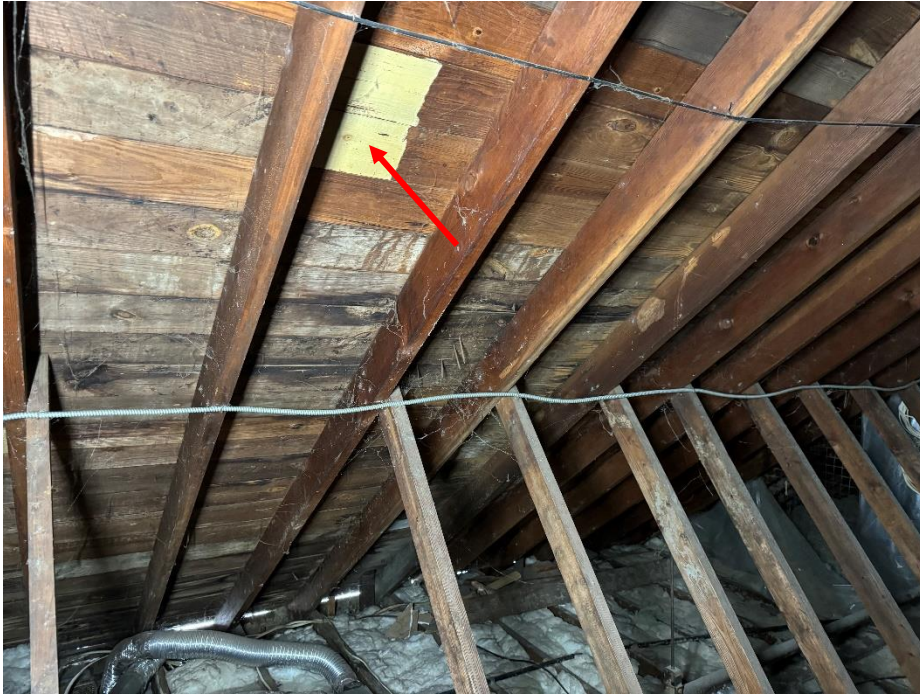
Photo 21. Bldg. 403 – Unit 1427: Red arrow pointing to coating applied on roof sheathing.
