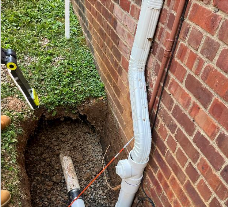
Photo 8 – Test Pit #3: Gravel encountered at bottom of test pit. Downspout attached to horizontal PVC pipe in test pit.
