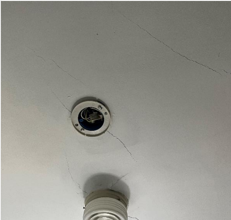
Photo 12 – Cracks in ceiling finishes of master bedroom of Unit 3202.
