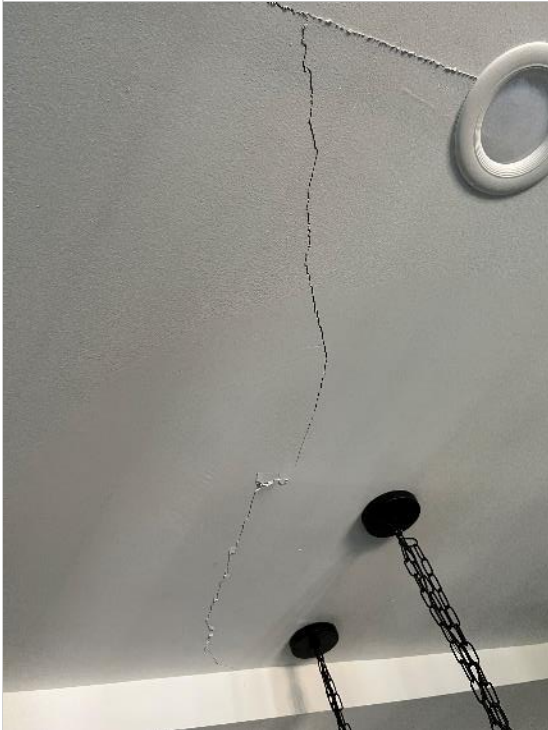
Photo 12 – Cracks in ceiling finishes of master bedroom of Unit 3202.
