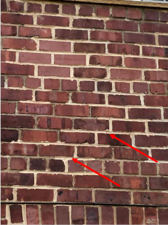
Photo 2 – Vertical sealant expansion joint in façade at rear elevation. Not previous repairs in façade adjacent to vertical expansion joint.
