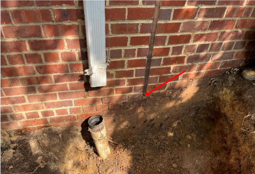
Photo 6 – Test Pit #1. Red arrow pointing to termination point of vertical sealant expansion joint. Note no waterproofing membrane and drainage board on exposed foundation walls.
