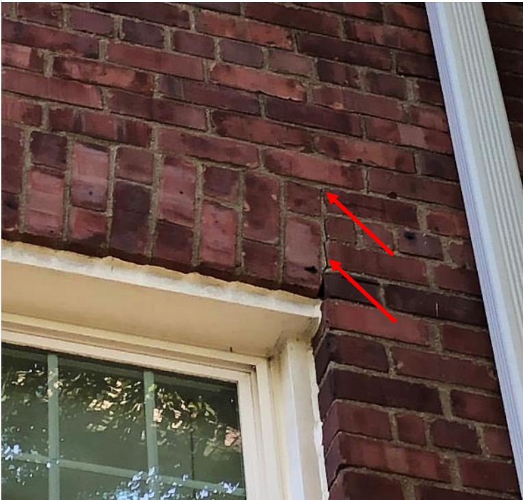
Photo 4 – Red arrows pointing to horizontal crack in brick lintel above window at rear elevation.
