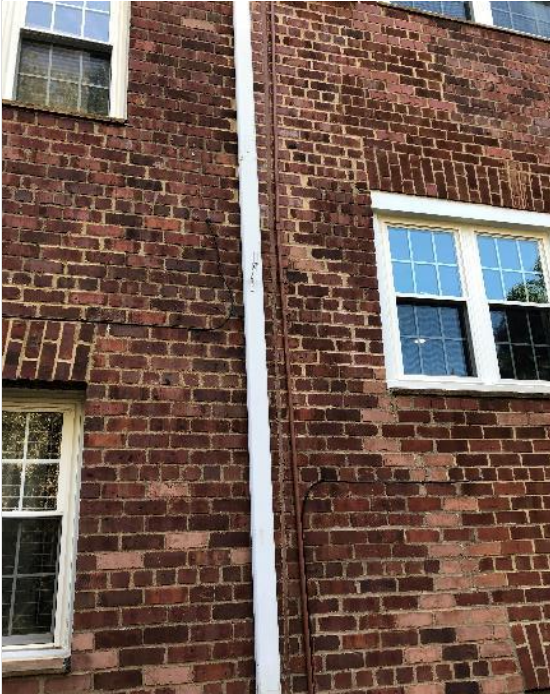
Photo 2 – Vertical sealant expansion joint in façade at rear elevation. Not previous repairs in façade adjacent to vertical expansion joint.
