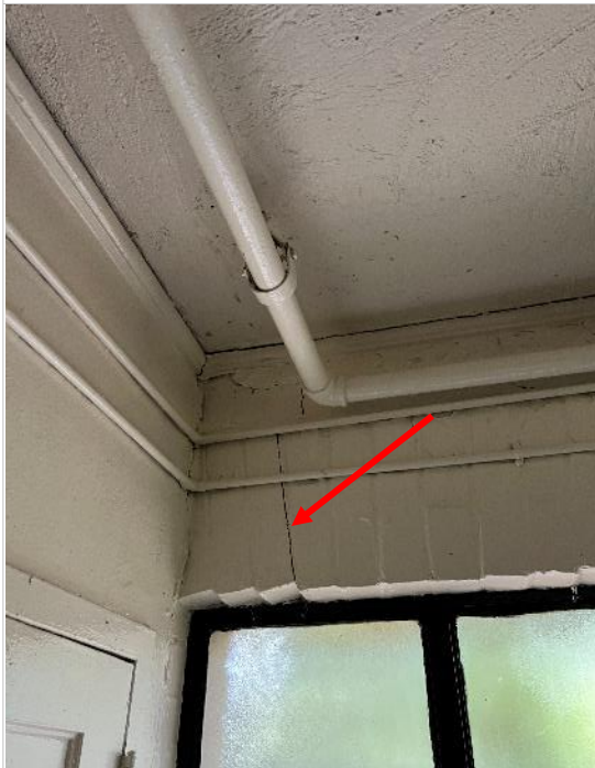
Photo 14 – Red arrow pointing to vertical crack in brick masonry above window from interior of laundry room.
