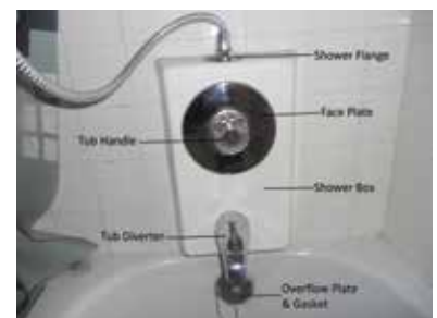
Diverter, Tub Handle, Overflow Plate & Flange: $117.00 (labor included)
