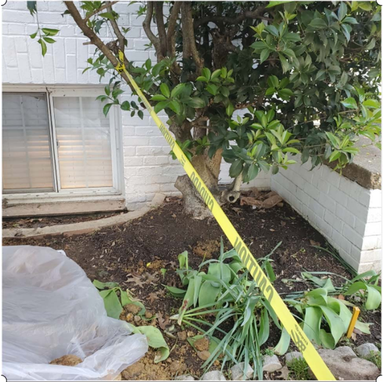
Left side of 1621's stoop—unable to dig behind the holly bush without damaging it to waterproof the wall because it is too close to the wall and they were told to not take out the holly bush.
