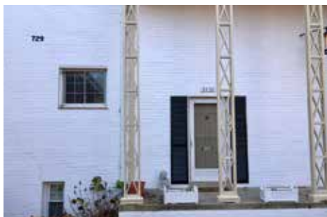
Under Contract in Days! 3436 Gunston Road
