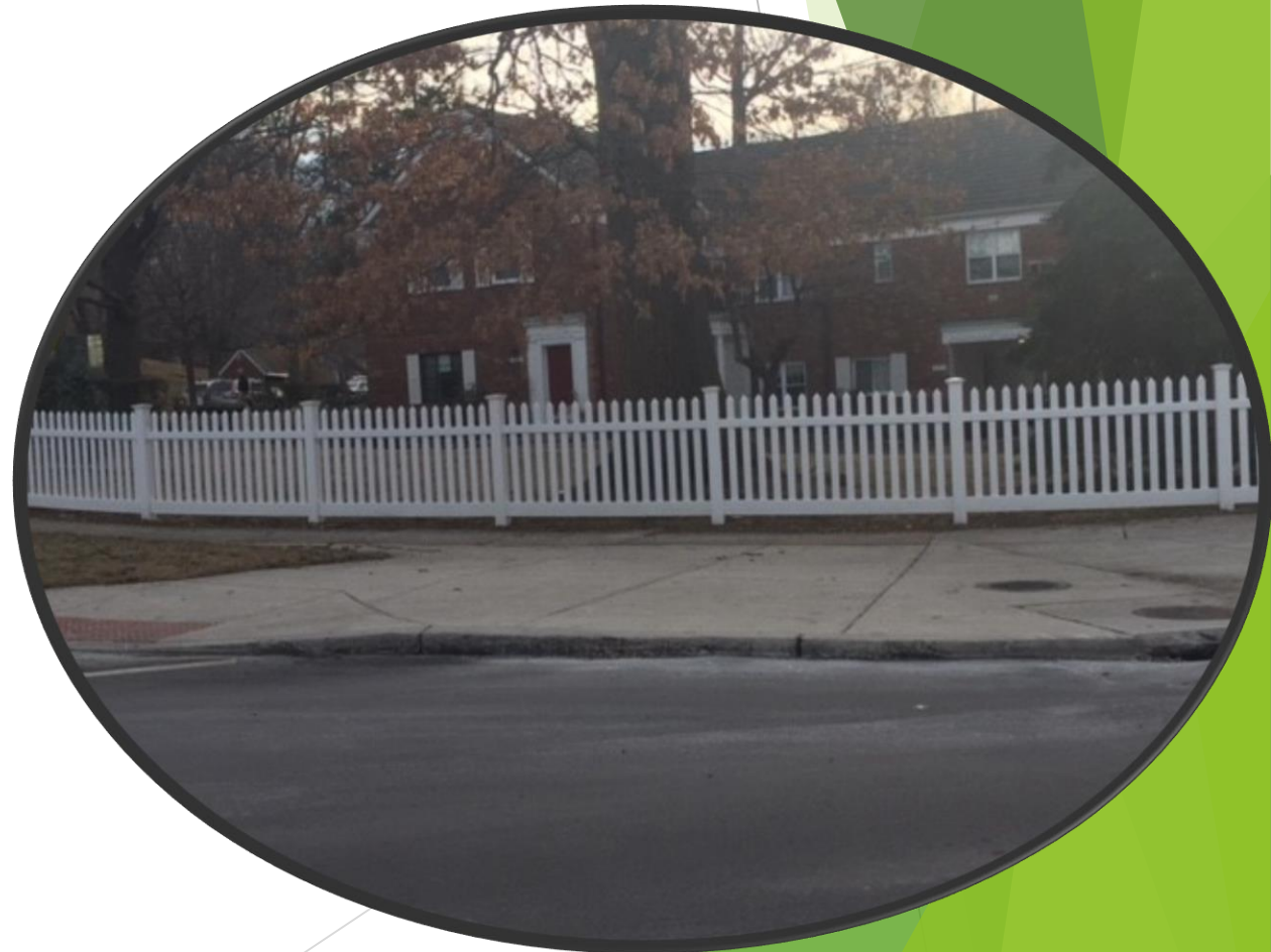
New fencing Valley cut through by 501
