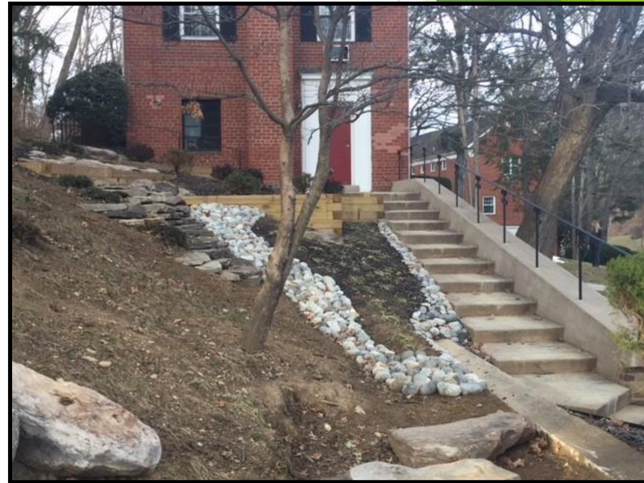
Slope Stabilization 944 Preston
