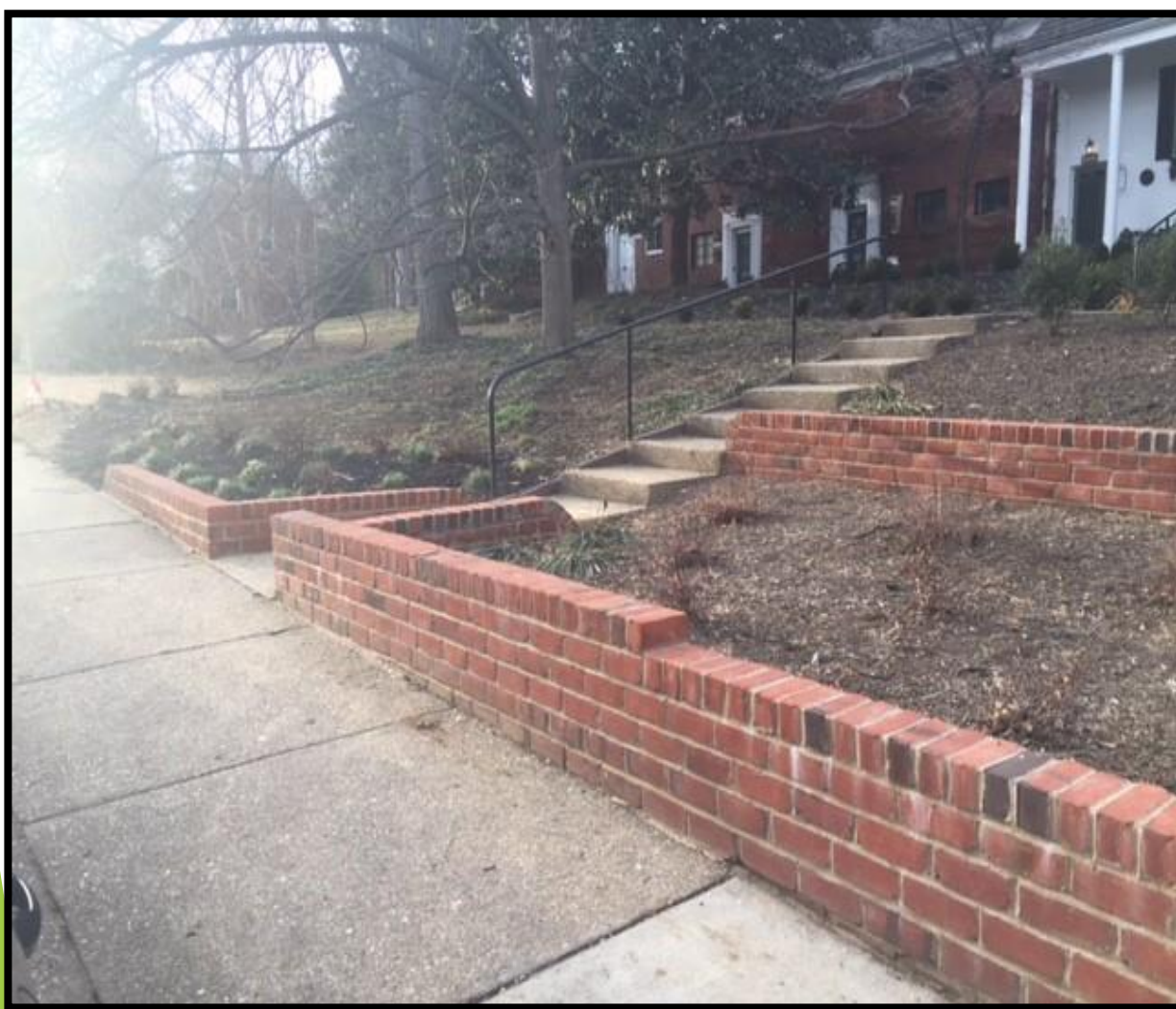
Slope Stabilization 948-950 Preston Road New Brick Walls and Beds
