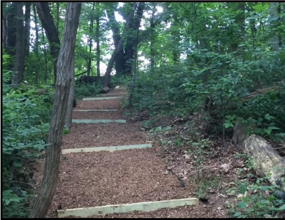
Newly restored path with water tables front of 701
